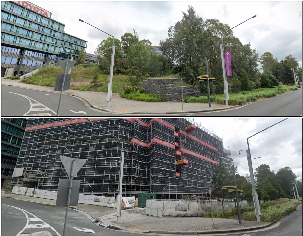
Figure 5: Imagery showing the original state of the land in December 2021 with mature vegetation, topography and gabion walls (top image) and the state of the land in October 2024 during construction works (lower image) (Source: Google Street View 2025).
